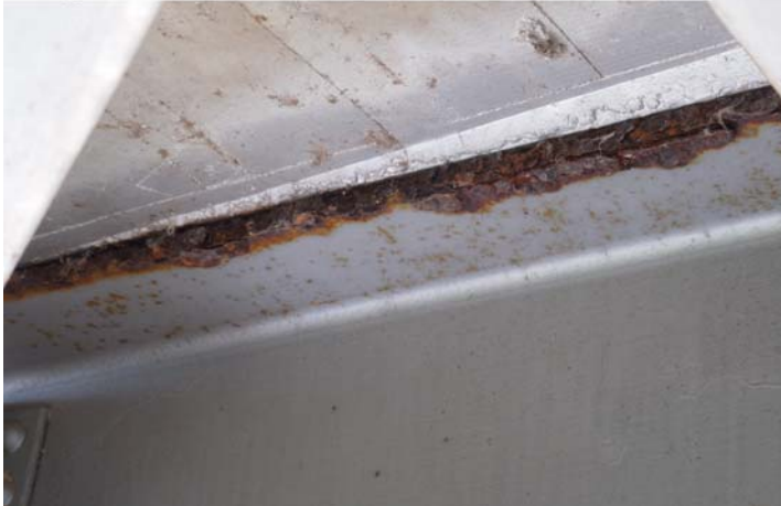
PP11, Lt: Corrosion and pack rust to the top flange of the floorbeam. Section loss to 3/16".
