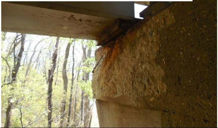
Bt 34, Bk, G1: Girder is slipping off bearing pad. Typical of G1 - G4 at this bent. Large spall with rebar exposed below bearing plate
