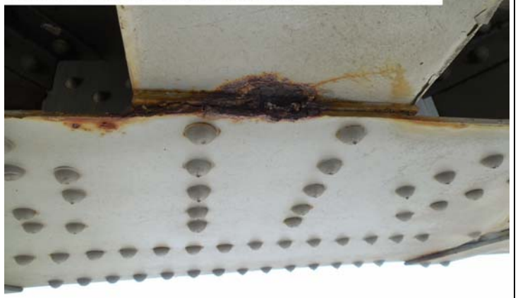
PP12, Lt: Section loss to the bottom flange of the floorbeam at gusset plate connection. Typical condition throughout.
