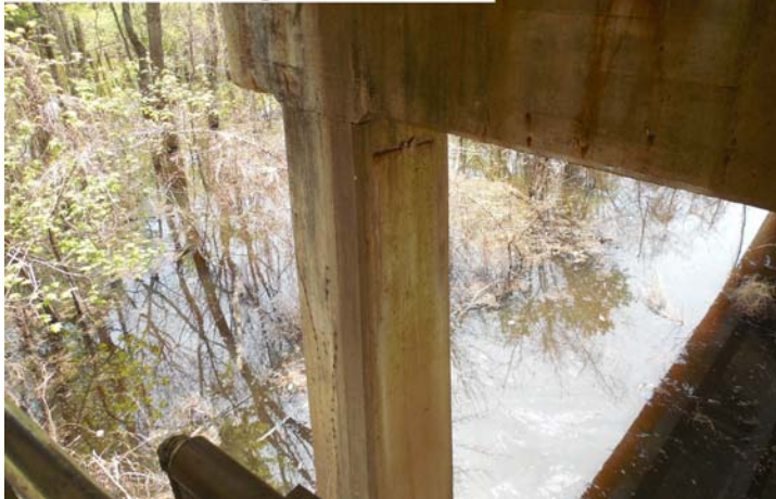
Bt. 49, Col. 1: Spalls with rebar exposed 1.5' long on side face.
