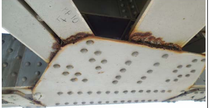
PP12, Lt: Section loss to the bottom flange of the floorbeam at gusset plate connection. Typical condition throughout.
