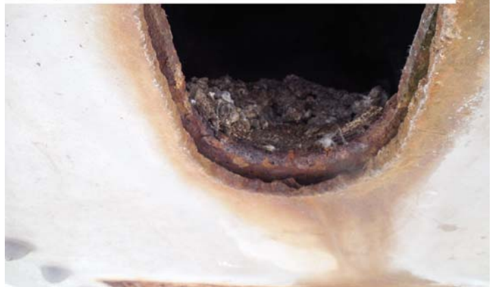
Bt. 55, Ahd: Cap has a 1' spall with rebar exposed.
