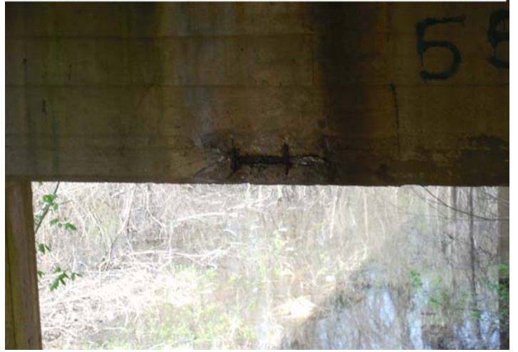
Bt. 55, Ahd: Cap has a 1' spall with rebar exposed.
