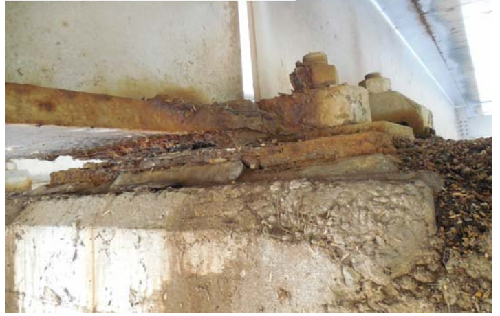
Bt 34, Bk, G1: Girder is slipping off bearing pad. Typical of G1 - G4 at this bent. Large spall with rebar exposed below bearing plate
