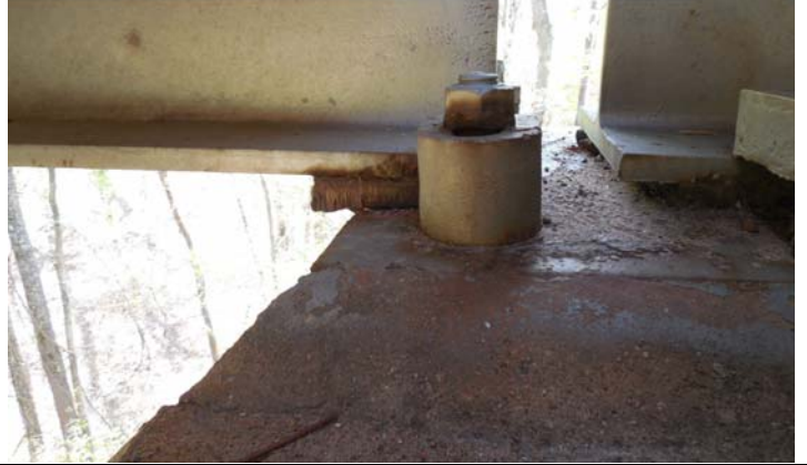
Bt 34, Bk, G1: Girder is slipping off bearing pad. Typical of G1 - G4 at this bent. Large spall with rebar exposed below bearing plate
