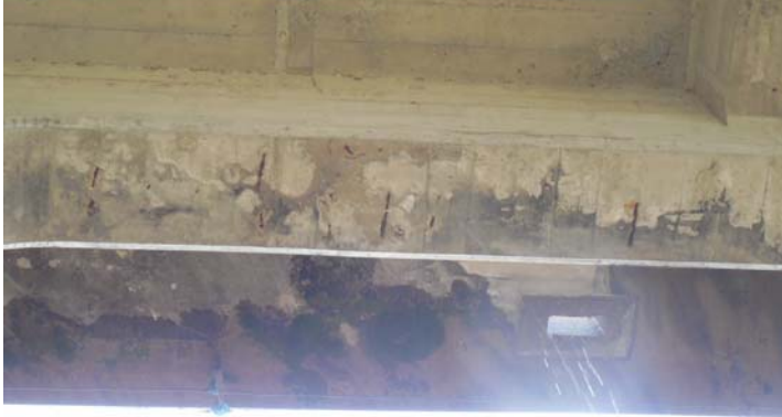
Span 16, Girder 1: Numerous shallow spalls with rebar exposed on bottom face.
