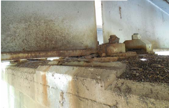
Bt 34, Bk, G1: Girder is slipping off bearing pad. Typical of G1 - G4 at this bent. Large spall with rebar exposed below bearing plate
